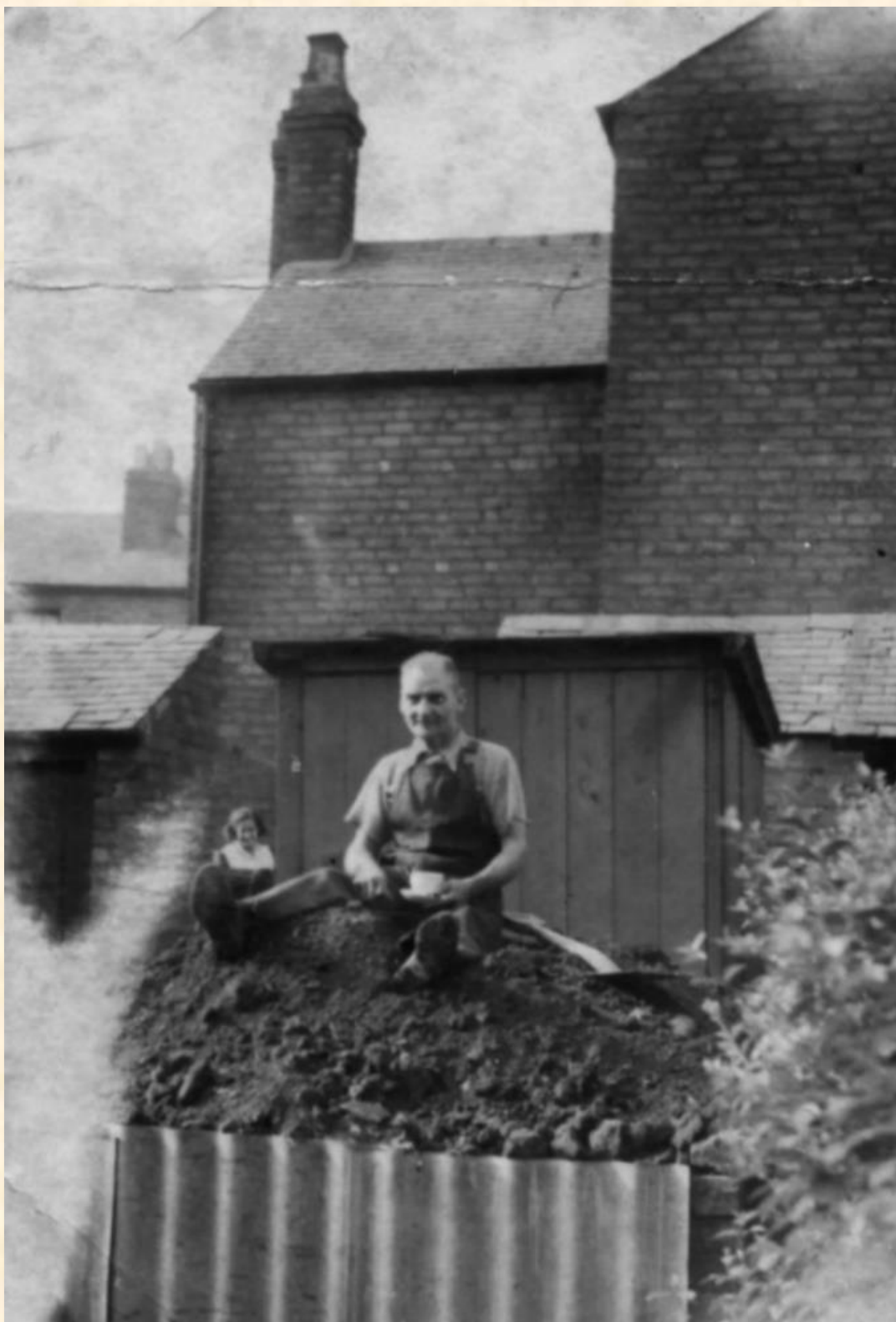
Arthur Clifford with the 'Anderson' air raid shelter he had just completed at 8 Roe Street, Derby. This was made from 14 panels and had a drainage sump in the floor to collect rainwater. According to the plans, Arthur had to dig a pit 4 ft (1.2m) deep, 4 ft 6 in (1.4 m) wide, and 6 ft 6 in (2.0 m) long. The shelter was 6 ft high, and Arthur covered the top 2 ft with the soil he had excavated. Internal comfort was up to him to devise. (With thanks to Arthur's granddaughter, Pat Carroll)
