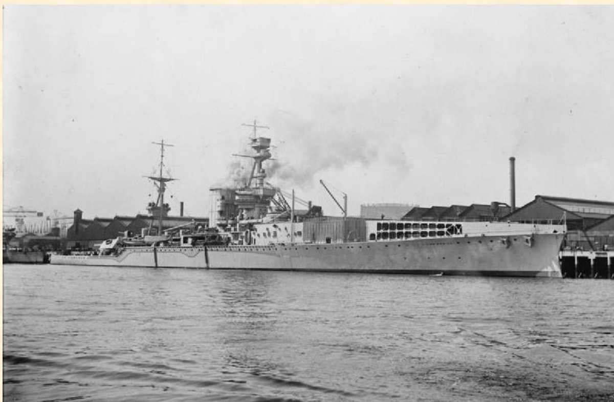
HMS Furious as originally completed in June 1917 by Armstrong Whitworth at their High Walker shipyard, just upstream from Jarrow. Note the flight deck forward of her bridge. My great grandfather, Charles Clifford, was a member of her first crew. She passed Jarrow on her maiden voyage into the North Sea in early July 1917. (Surgeon Parkes Collection; © Imperial War Museum, ref. SP89 )
