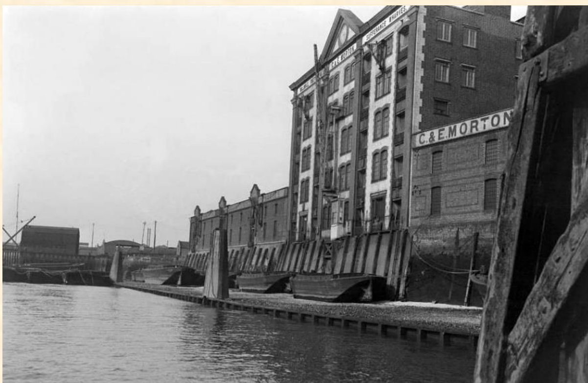
C & E Morton Ltd's food preservative factory at Sufferance Wharf, Millwall, on the bank of the Thames on the west side of the Isle of Dogs, seen here in the early 1930s. Susan's son, John, worked for the company and its later owners for many years. (Photographer – A G Linney, Port of London Authority; Museum of London Docklands Collection )
