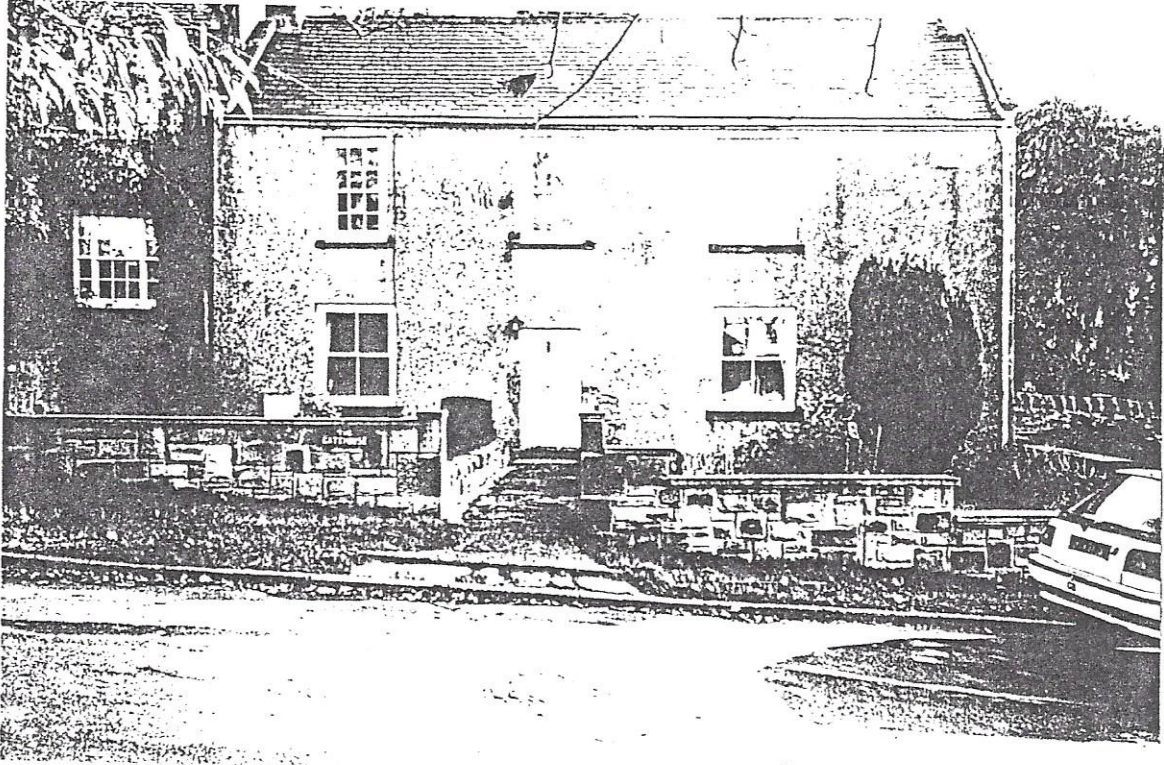
Plate 16: Tanfield: The Gate House.
